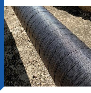
Polyguard's RD-6® Coating System is a non-shielding anti-corrosion system used on buried and submerged line pipe, rehabilitation and new construction girth welds. RD-6® can also be used above ground but the coating must be protected from harmful UV rays.
