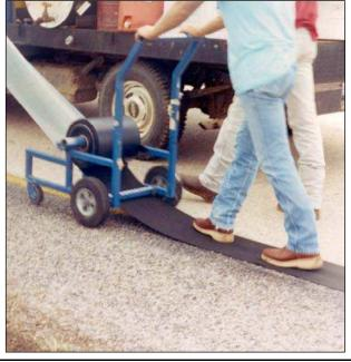
"...waterproofing membranes have reduced the rate of reflective cracking...even when reflective cracking appears over joints with membrane treatment, the cracks appear to stay tighter than cracks over joints without membrane treatment."
