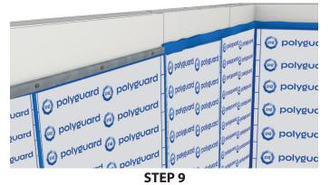
All Home Stretch 40 Mil Membrane wall terminations shall receive a termination bar (supplied by others). Firmly press the termination edge with a hard, narrow, hand-held roller; install the termination bar with fasteners, and then cover the membrane edge and termination bar with a tooled bead of Blue Barrier Gap Filler as a termination protection.
