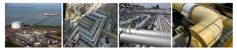
**Insulrap**<sup>m</sup> **JB** is a self-adhesive multi-layer white PET/FOIL/PET zero perm membrane designed specifically for LNG and Cryogenic insulation systems. The product is constructed of a proprietary Polyguard butyl compound, which is a peel and stick self-sealing with excellent low temperature adhesion and flexibility.
