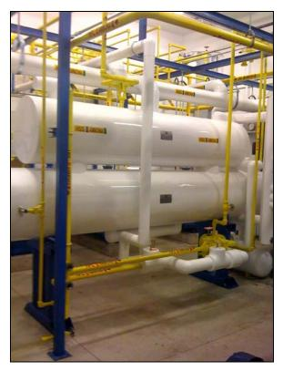
**Alumaguard®** Lite White flexible weatherproofing cladding from **Polyguard Products** is the newest member of the **Alumaguard®** family of cladding products that offers indoor/outdoor installation, superior cold weather performance, enhanced chemical resistance, ease of handling and application and true zero perm performance
