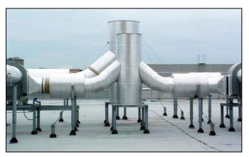
**Alumaguard** should not be adhered directly to commercial roofing membranes. For specific information regarding **Alumaguard** and commercial roofing, refer to Technical Bulletin, 2011-1.
