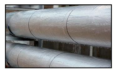
**Alumaguard**® (formerly Alumaguard® 60) weather-proofing cladding from **Polyguard** products is the original, flexible self-healing membrane used world-wide on exterior ductwork, refrigeration and chilled water piping, tanks, vessels and equipment.
