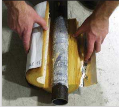
Figure 11: Reactive Gel Applied to Pipe
