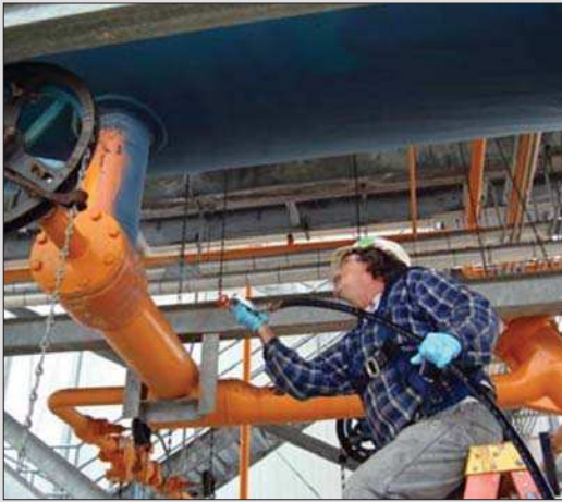
Figure 4: Gel Being Spray Applied
