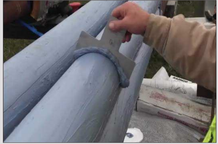
Figure 3: Using Calibrated Trowel to Apply Gel
