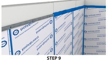
All Home Stretch 40 Mil Membrane wall terminations shall receive a termination bar (supplied by others). Firmly press the termination edge with a hard, narrow, hand-held roller; install the termination bar with fasteners, and then cover the membrane edge and termination bar with a tooled bead of Blue Barrier Gap Filler as a termination protection.
