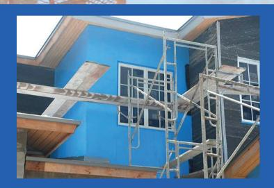
Blue Barrier™ Liquid Wrap 2300 is a low VOC spray applied, fully adhered, permeable, air and moisture building envelope protection membrane. This thin mil, seamless substrate coating can be applied with an approved airless sprayer or power rolled. Liquid Wrap can be sprayed over clean and debris free surfaces and substrates such as OSB, plywood or exterior gypsum.
