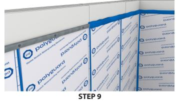
All WM40 wall terminations shall receive a termination bar (supplied by others). Firmly press the termination edge with a hard, narrow, hand-held roller; install the termination bar with fasteners, and then cover the membrane edge and termination bar with a tooled bead of Blue Barrier Gap Filler as a termination protection.
