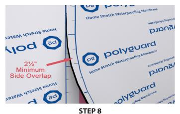
WM40 side laps shall be 2-1/2 inches minimum. Staggered end laps shall be 6 inches minimum.
