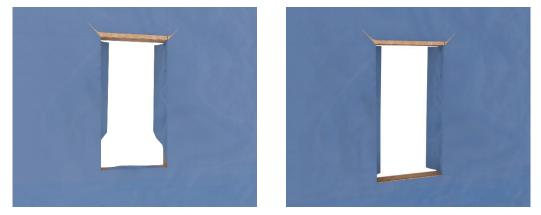
STEP 4 - Option ASTEP 4 - Option BOn the vertical side of the window fold the WRB back past the jamb and tack it there. Using<br/>your utility knife cut the WRB at the middle of the jamb. Then tape this WRB in place with a<br/>3-inch contractors/housewrap tape. This allows for a sealing or termination of the WRB.
