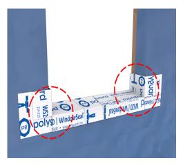
STEP 8 Cut flashing patches of WS20 and install at each of the sill corners.
