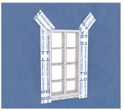
STEP 14 Cut 2 sections of WS20 6-inches to cover the 45-degree cuts in the WRB.
