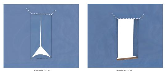
STEP 3A STEP 3B At top of the WRB horizontally cut with a utility knife from edge to edge. At each of the top corners cut the WRB at a 45 degree angle roughly 6-inches heading away from the window.
