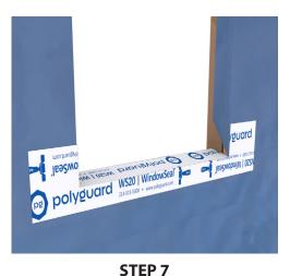
Cut at the corners of the rough opening so that the WS20 may be folded onto the WRB surface.
