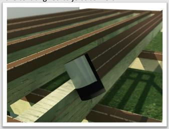
**3.** Pull split release liner to halfway point and adhere one side, smoothing by hand, then pull the remaining 2" of the liner and hand-smooth tape to joist.
