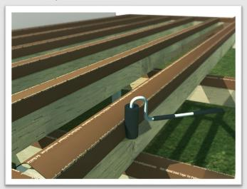
5. Roll over the entire surface using a hand roller, smoothing the tape and boosting the bond of adhesive to joist surface
