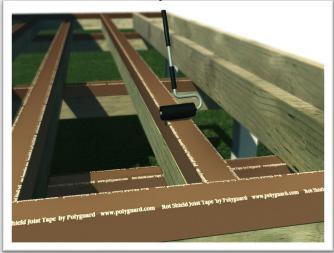
**6.** Complete job, laying deck boards. Rot Shield Joist Tape is brown so will camouflage well beneath deck boards.
