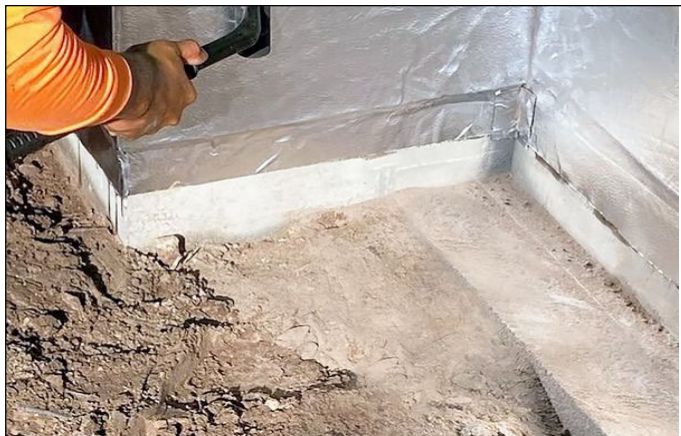
TERM FUV Flashing|Termite Barrier is also available with aluminum foil UV resistant backing, offering up to 12 months UV resistance. Available widths are 12" and 18".
