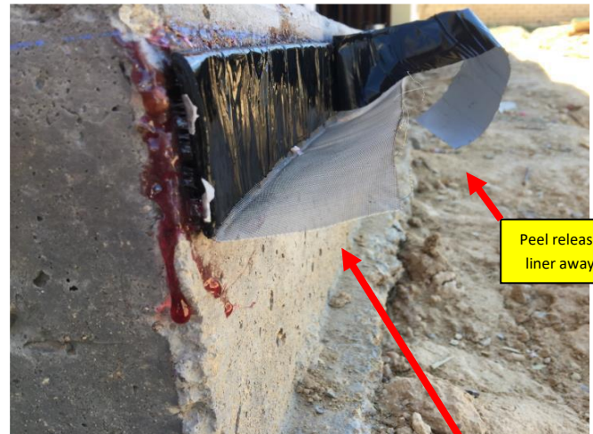
TERM ™ Isolation Joint Barrier installed on a Waco, TX residence. The barrier is adhered to the side of the house slab. Prior to driveway pour, release liner is removed and 0.018” Micromesh screen is folded out to horizontal. The result is a termite barrier embedded in the concrete.
