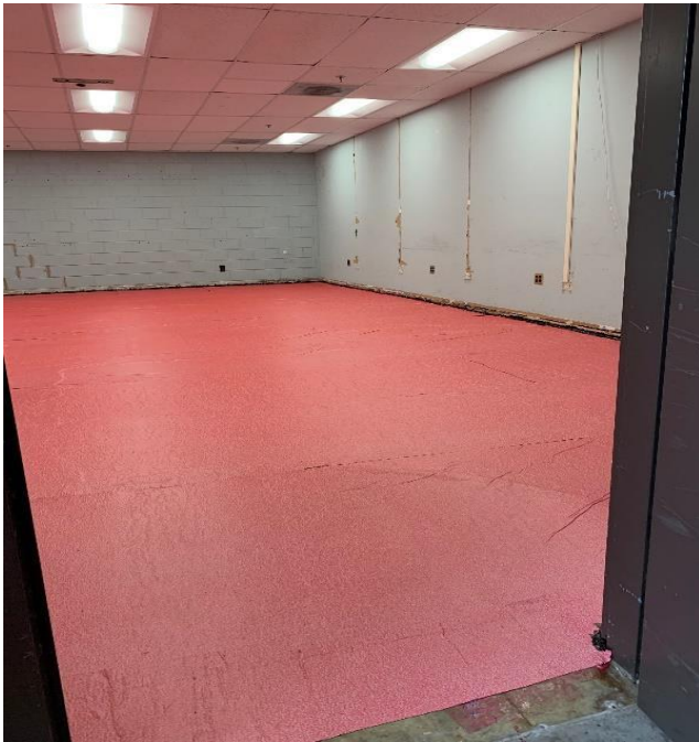
TERM® Wood Floor Underlayment Vapor and Termite Barrier
