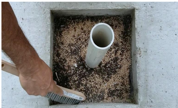
Clean cavity including walls to prevent termite access
