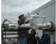
**Tanks & Vessels:** Insulating tanks and vessels is similar to piping where single and double layering patterns of insulation should be followed. Joints should be overlapped by 6" on centers. Joint sealant to be applied to the outer layer. Use filament tape or metal banding to hold insulation tightly in place.
