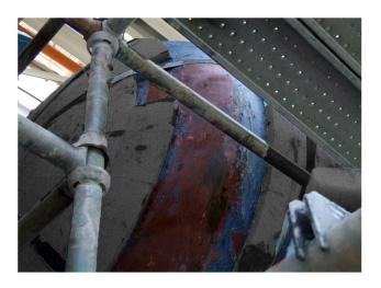
**Head Installation:** Heads to be fabricated and form fitted. To be applied in sections. RG will help adhere insulation to tank heads and bottoms.
