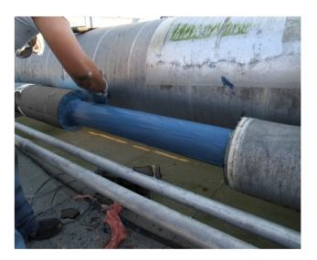
In the illustration above (left) moisture got caught inbetween the pipe and insulation. The epoxy paint was not able to prevent corrosion. Rigid paint type coatings can crack as pipes expand and contract. Because it remains flexible, reactive gel is better suited to flow with the pipe and not chip or flake off, allowing corrosion to occur.
