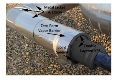
**Pipe Protection:** It is highly recommended on cold systems to install cathodic protection to piping under insulation. No matter how good the insulation and jacketing is, over time moisture will get caught inbetween the pipe and insulation.
